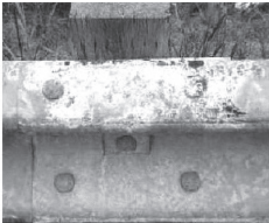
Figure 3.23 Corrosion at the joints
