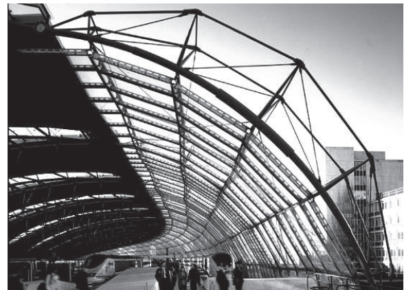
Figure 7.32 Waterloo International Terminal Western side view of the concourse
