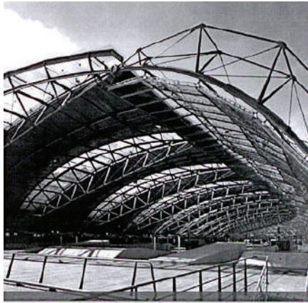
Figure 7.31 Waterloo International Terminal Roof design
