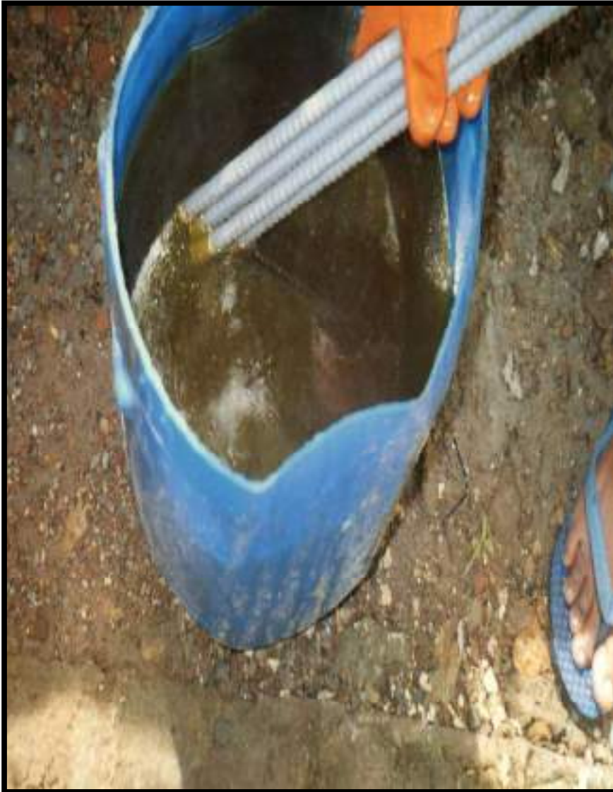
Rust Removal – Acid Pickling
