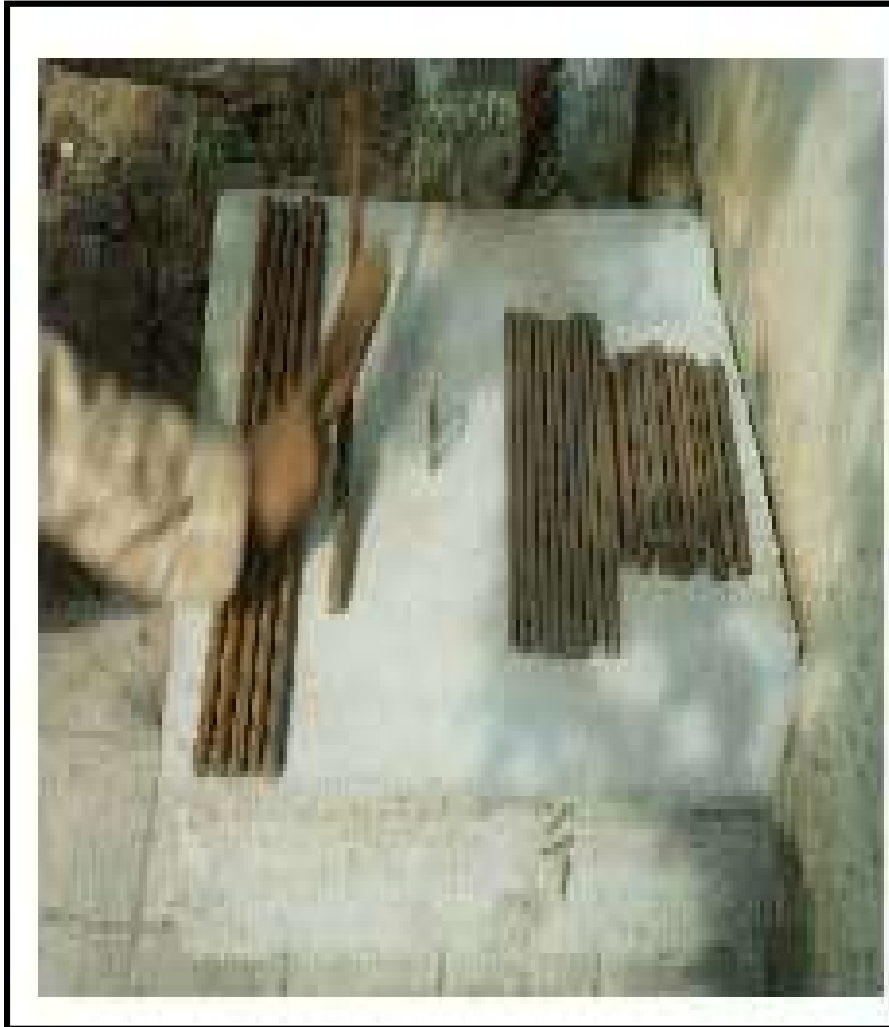
Loose Rust Removal – Steel Wire Brush Cleaning
